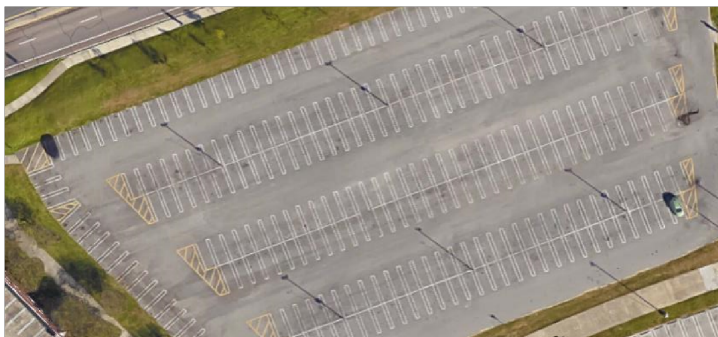
Lot D2 Parking Area
