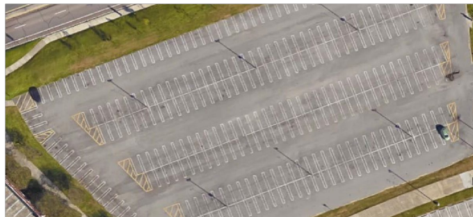
Lot D2 Parking Area
